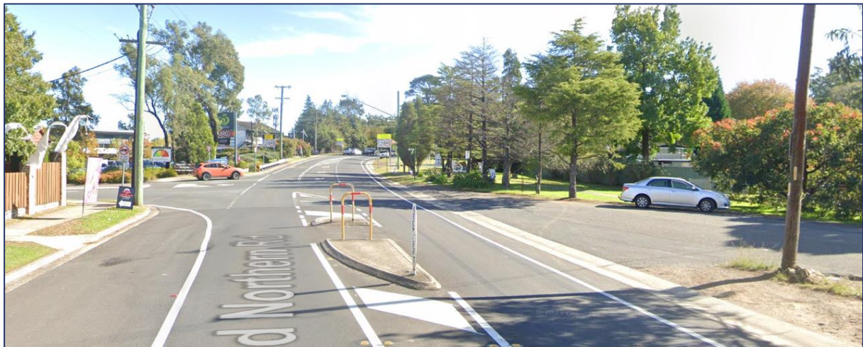
Figure 6: Old Northern Road Pedestrian Refuge
